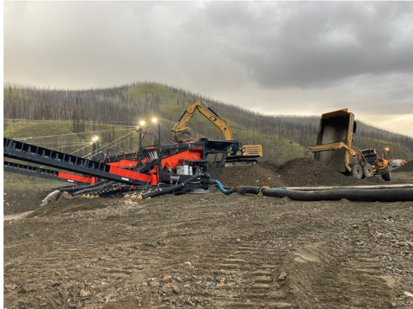
Fig. 1 – Paygravels hauled by Truck and fed by Excavator into two parallel Washplants equipped with Drag Chain Feeders
